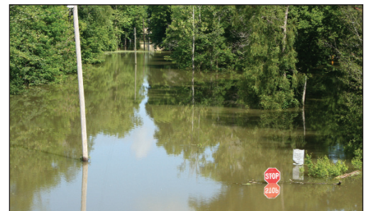
Backwater County Road underwater
