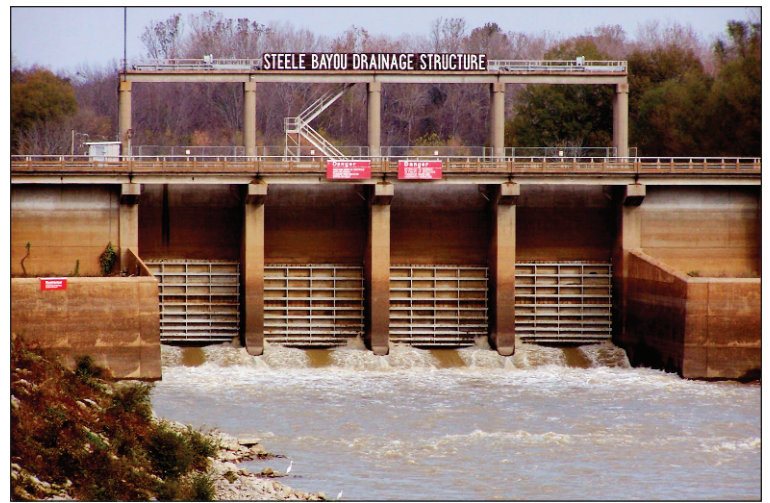
Steele Bayou Structure
